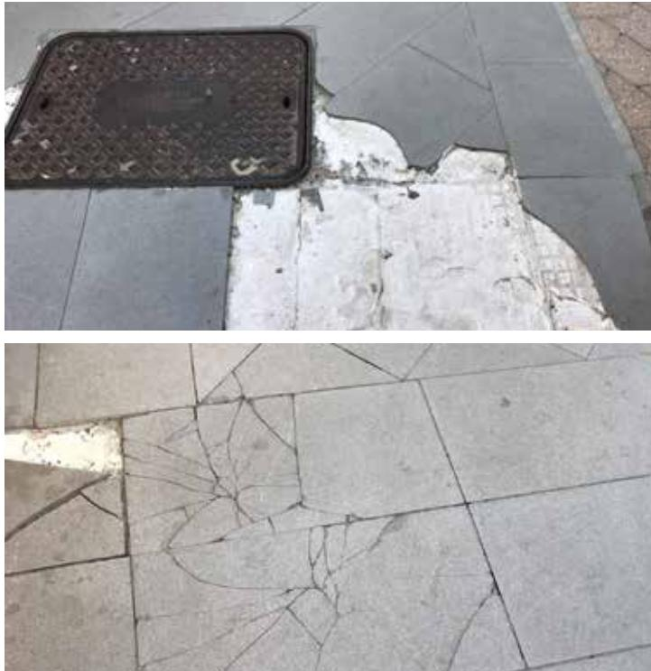
Paving with increased thickness to 2 cm guarantees high mechanical and resilience (ability to absorb shocks) properties, to avoid any breakages due to the inability to take heavy loads, such as vehicle crossing and stresses caused by temperatures below zero. These inabilities are typical for pavings with lower thickness. Therefore, L'Altra Pietra is the perfect paving for many different uses in outdoor environments.
