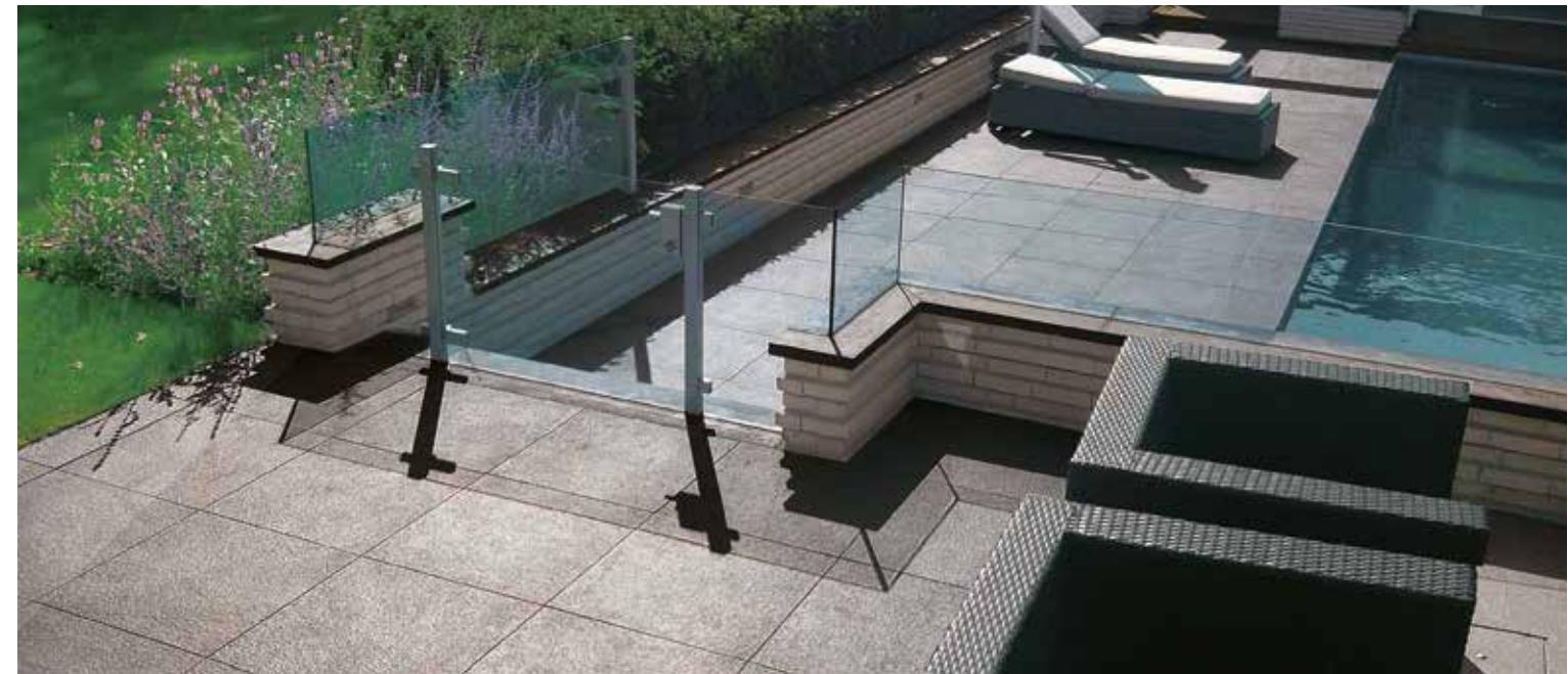
The advanced technical features of thick Granulati Zandobbio collections, combined with an adhesive laying technique on screed, allow users to create perfectly stable and exceptionally hard-wearing surfaces. Granulati Zandobbio slabs used with this solution can withstand both moving and parked vehicles. Ideal for heavily frequented areas, particularly for squares, pavements, or ramps.
